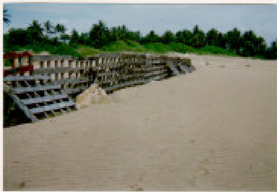
Sand fence at Barceloneta, Puerto Rico 1996
